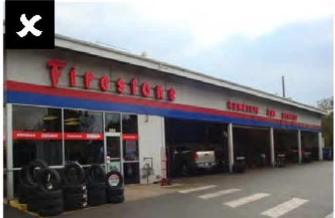
Service bays on primary facade
