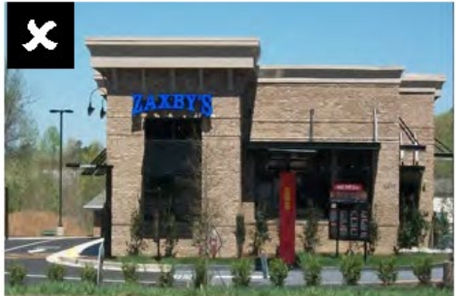
Drive-through ordering station on primary facade
