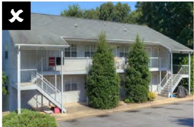
Exterior stairs and circulation corridors
