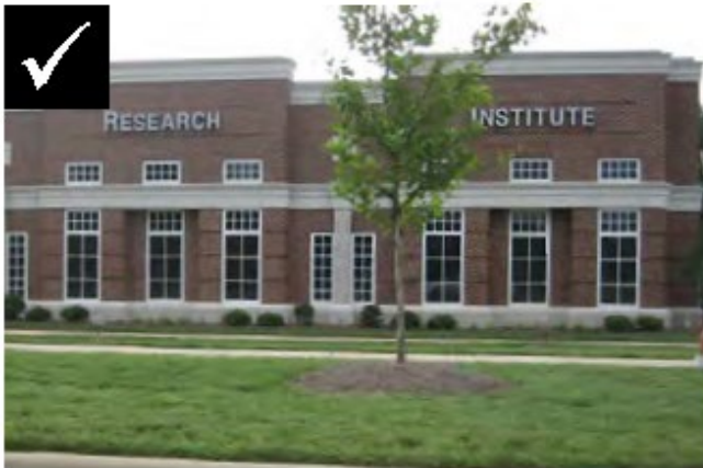
Continuous parapet with height changes
