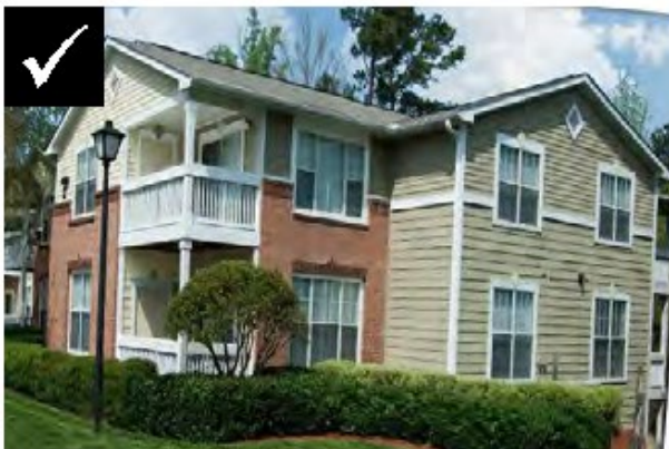
Adequate windows with regular rhythm and alignment
