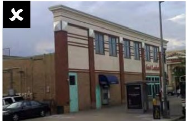
Non-continuous parapet without height changes
