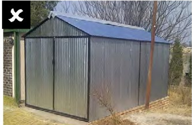
Materials do not match principal structure
