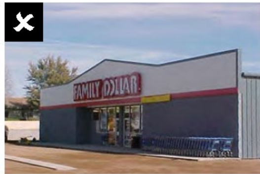
Painted concrete block and metal facades
